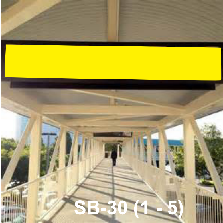
Level 2 Oversight Bridge - West Concourse to Hyatt
